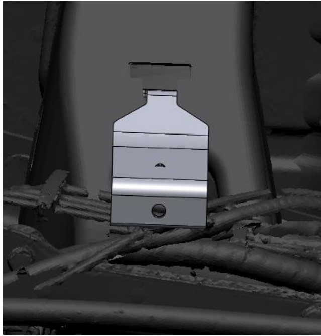
Installed A Tab Strap for Front Support.
