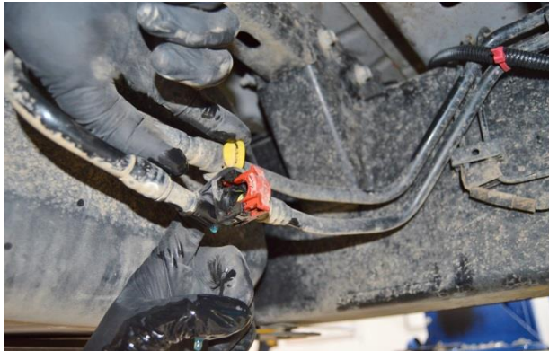
(Fig. 5) Fuel line connectors at front of tank.
