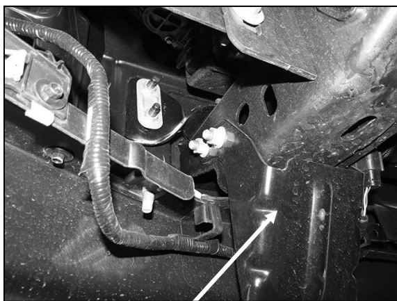
(Fig 8) Driver/left frame extension pictured
