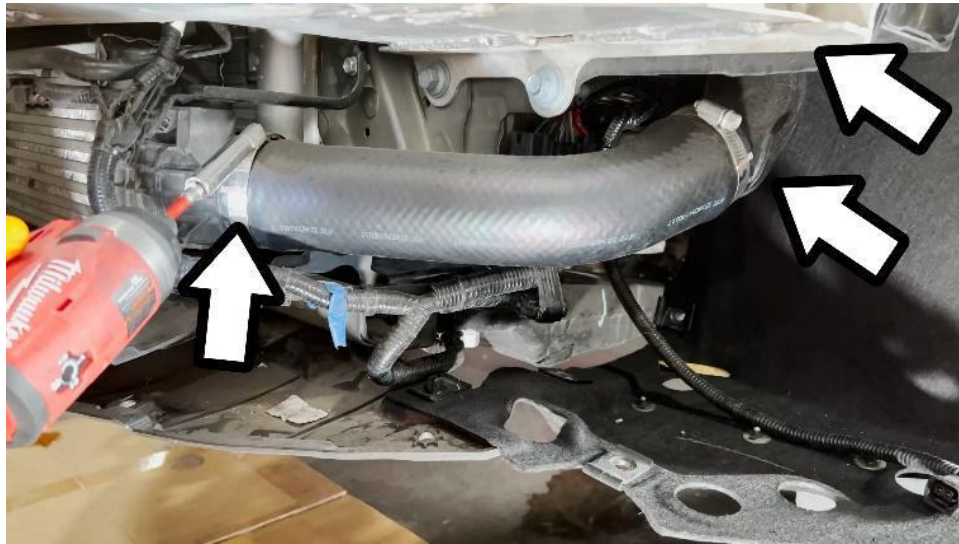
15. Loosen the hose clamp securing the charge hose from the intercooler. Remove the 10mm bolt securing the factory charge pipe bracket from the inner wheel well. Loosen the hose clamp securing the resonator hose from the charge pipe.
