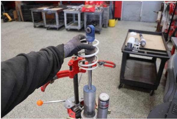
Step 9. Remove tender spring.
