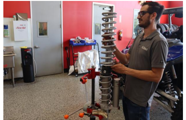
Install the Eibach rear main spring and compress the springs.
