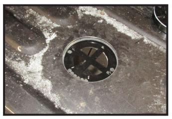
Using the provided template, mark pilot holes and slots. Drill pilot holes as marked.
