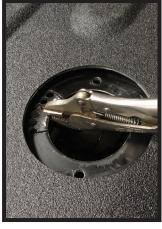
Using a reciprocating saw, cut the marked notches out. Using a pair of visegrips, remove the metal notch.
