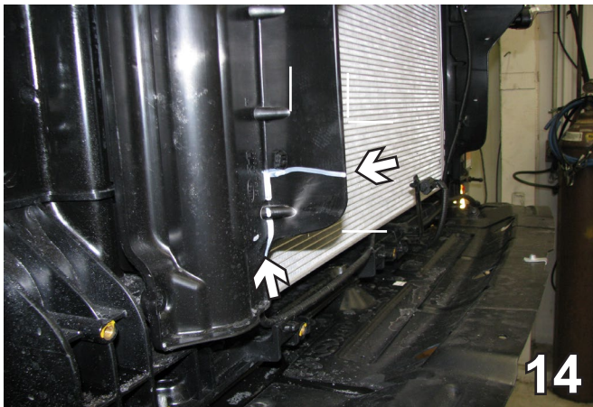
14. Trim on the inner edge of the air dam, under the grommet and cut straight down the crease. Remove this area with the reciprocating saw, both sides.
