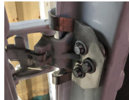
Figure 5: Inside View of Installed Upper Hinge
