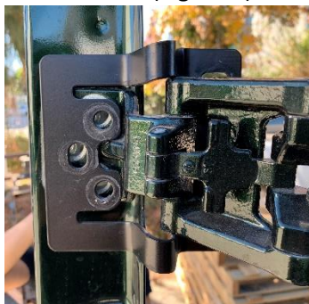
Figure 3: Bracket Installed Over Factory Hinge
