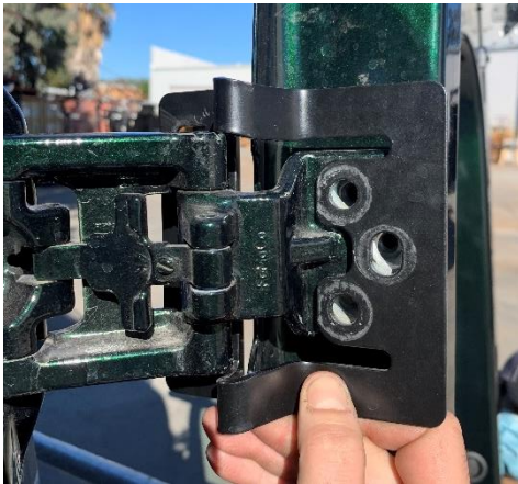
Figure 3: Bracket Installed Over Factory Hinge
