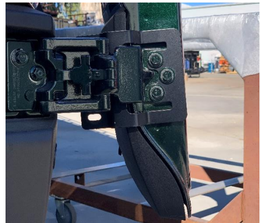
Figure 4: Inside View of Installed Lower Hinge Bracket
