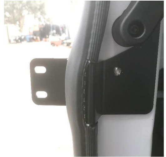
Figure 15: Installed Weather Stripping After Modification
