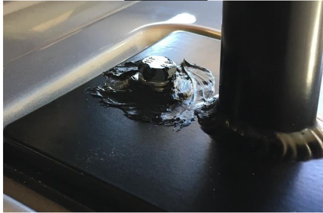
Figure 5: Final Silicone Seal
