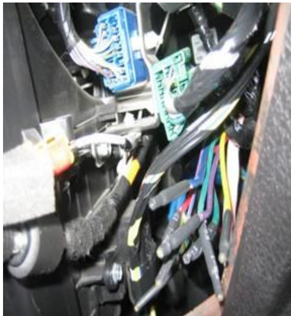
View looking through glove box opening
